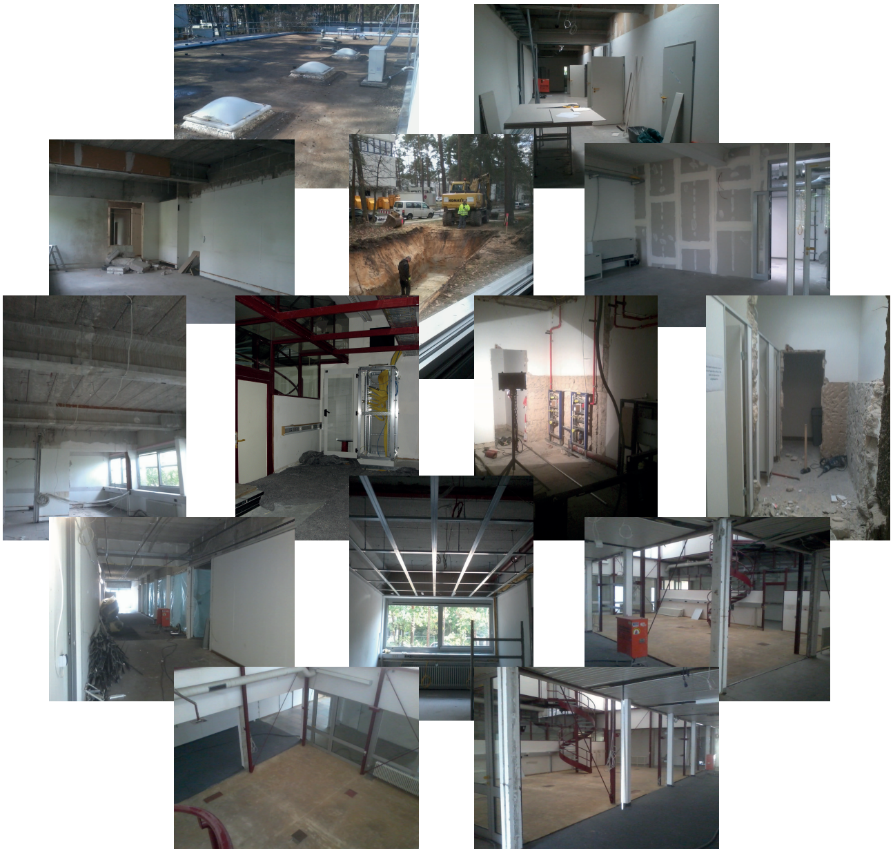
Figure 1: Some images of the LTM-building taken during construction project
